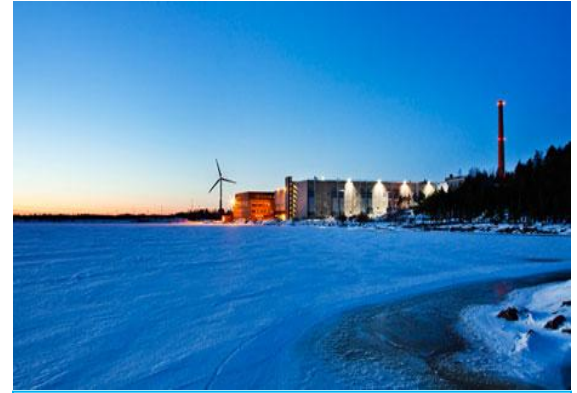
Google's data centre in Hamina, Finland, where the company has renovated an old paper mill to take advantage of the building's infrastructure and its proximity to the Gulf of Finland's cooling waters. Photograph: Google
