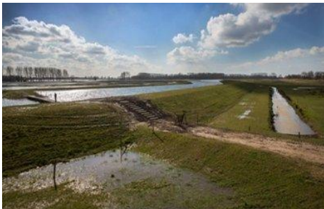
The Noordwaard polder in Werkendam is one of the key areas of the national Room for the River project. Photograph: Courtesy Werry Crone / Noordwaardpolder RR project
