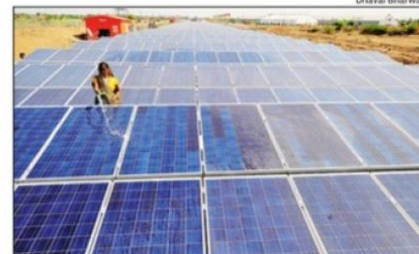
SILICON VALLEY: Solar panels on the Narmada canal in Gujarat generate power while reducing evaporative loss of water
