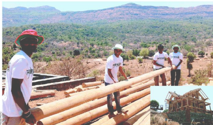
A log house, imported from Russia, is being assembled in India by Russia-trained Indian workers.
