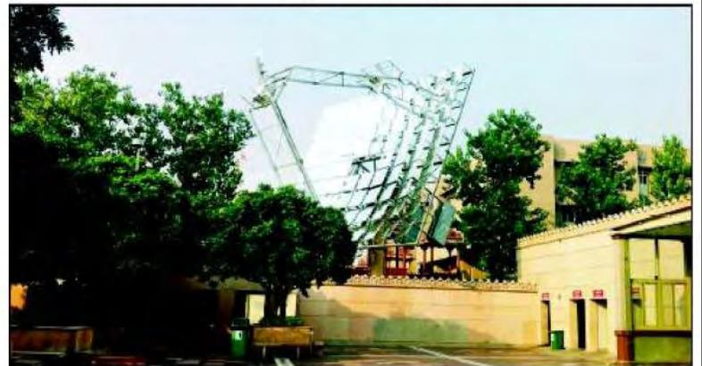
BRIGHT IDEA: The solar concentrator at the temple produces steam which powers the cooking procedure
