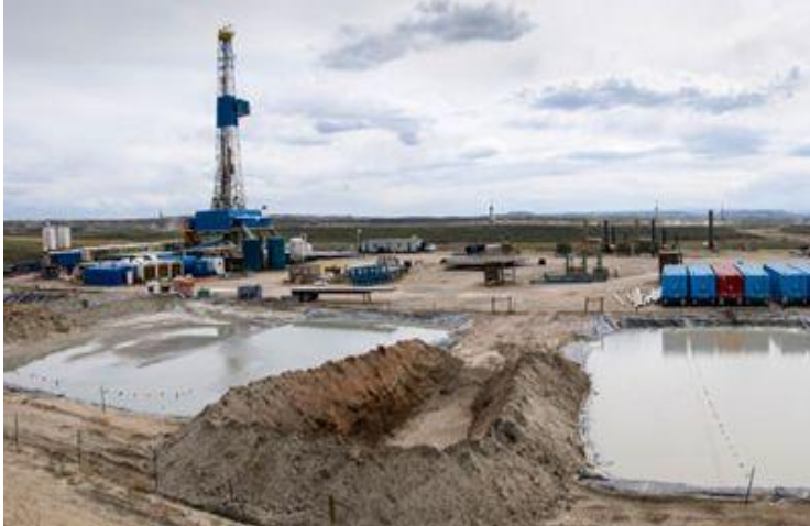
Wastewater evaporation pits from gas drilling and fracking in Pinedale area in Wyoming. Photograph: Ted Wood/Corbis
