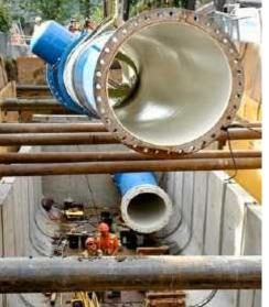
Installing LucidPipe technology, which uses gravity to generate energy. Photograph: Sherri Kaven
