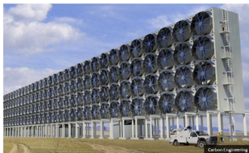
Carbon Engineering's technology for capturing carbon dioxide from ambient air involves giant air-sucking modules that separate out the CO 2 and put it into a solution for recycling into usable gas
