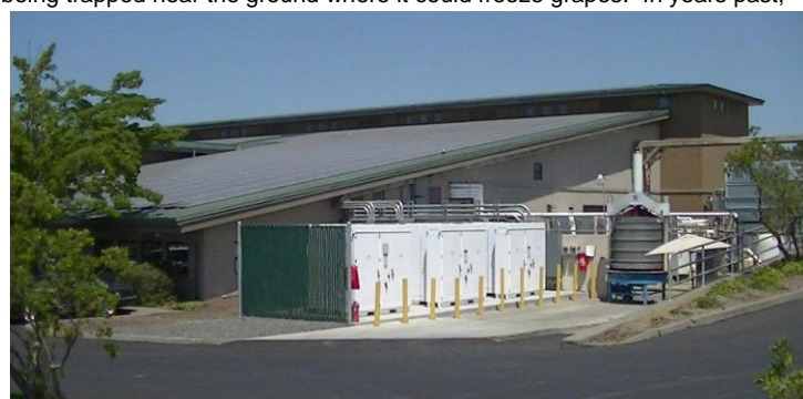
Solar panels line the rooftop of the La Crema winery and provide most of its power. Outside, newly installed Tesla batteries store excess solar generated electricity for later use.
