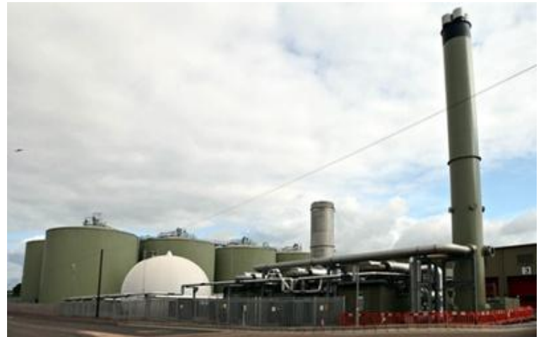
Food waste from Sainsbury's supermarkets around the UK is delivered by lorry to Biffa's plant in Cannock, and turned into bio-methane gas which is then used to generate electricity. Photograph: Diensen Pamben/Getty Images
